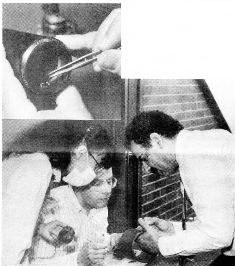
Michael Khanchalian gave a Wax Cylinder Repair Workshop. In this photo he demonstrates the proper technique for filling pits in a concert cylinder to Anna-Maria Manuel and Bill Klinger. Inset, above center: Here Mike demonstrates how to repair a crack in a cylinder. He heats a small metal staple over an alcohol lamp and allows it to "drop" into the wax, but not to penetrate through the groove surface. The temperature of the staple is critical.
